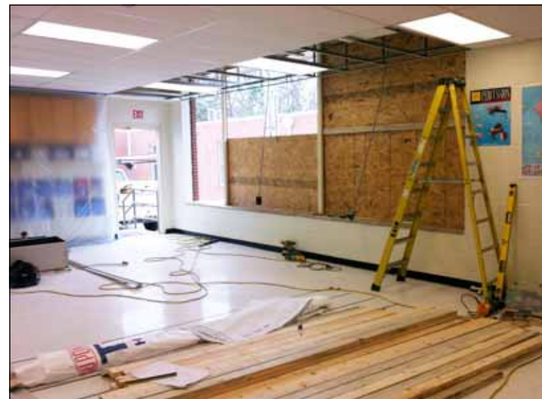
Windows being replaced in an SES classroom. Photo by Pagie Wilson
